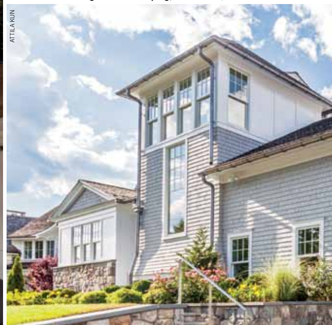
A different house in Old Greenwich—this one still available to some lucky buyer—walked away with the HOBBI for Best Spec Home $5 Million–$6 Million. PROJECT TEAM: Builder: Karp Associates, New Canaan; Architecture: Jones Byrne Margeotes Partners, Greenwich; Landscape design: T.R. Molgrano Landscaping, Stamford ↓
